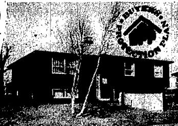
Looking for low utility bills — this home is extremely well insulated. Siding never needs painting. Take a look and see all the benefits this home can offer your family.
